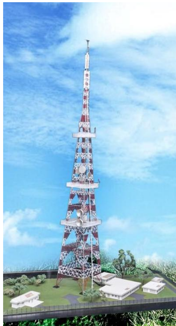
Figure 2 : Kokavil Transmission Tower
