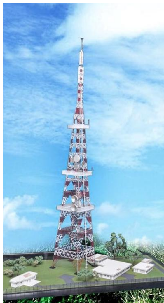
Figure 2 : Kokavil Transmission Tower
